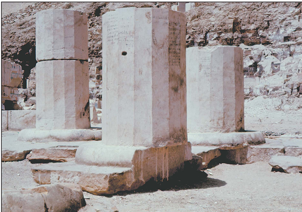
Remains of the colonnaded hall in the Tuthmosis III temple at Deir el-Bahari (Photo J. Lipińska's archives)
