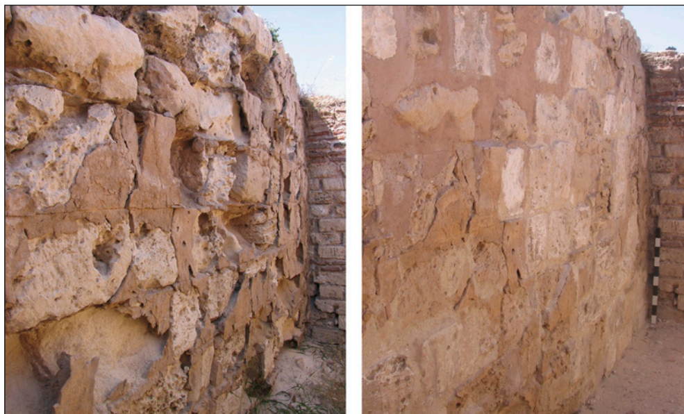
Fig. 22. North wall of the cistern: left, before, and right, after conservation (Photos G. Majcherek)
