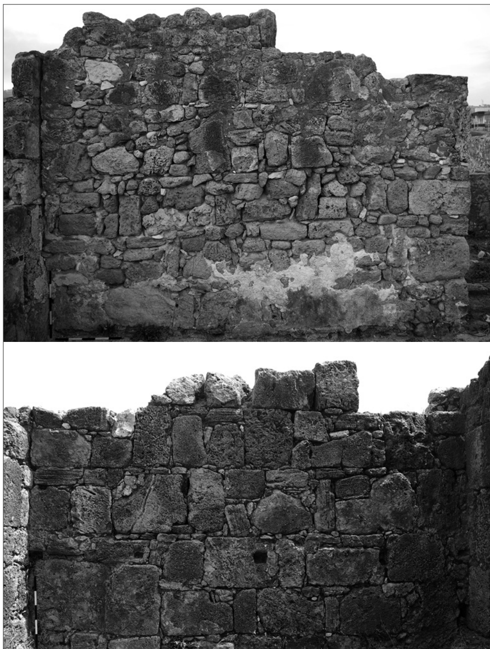
Fig. 4. Examples of wall bonds: top, south wall of area 25; bottom, east wall of area 22 (Photos M. Dzik)
