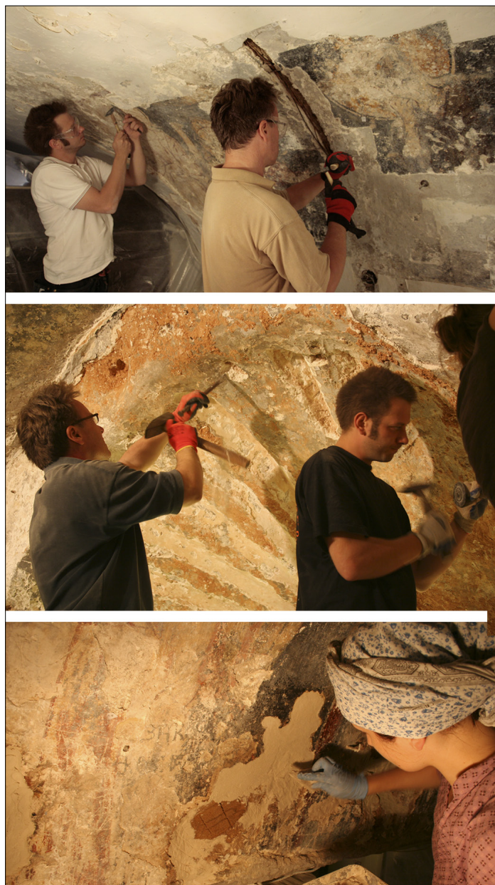
Fig. 3. Uncovering the wall paintings in the presbytery of the Mar Elias Btina church: top, removing plaster coats from paintings on the north wall; center, removing non-original plaster from the conch (discernible shape of the carved shell decoration); bottom, new mortar filling gaps in the murals on the south wall (Photos M. Rogowska)
