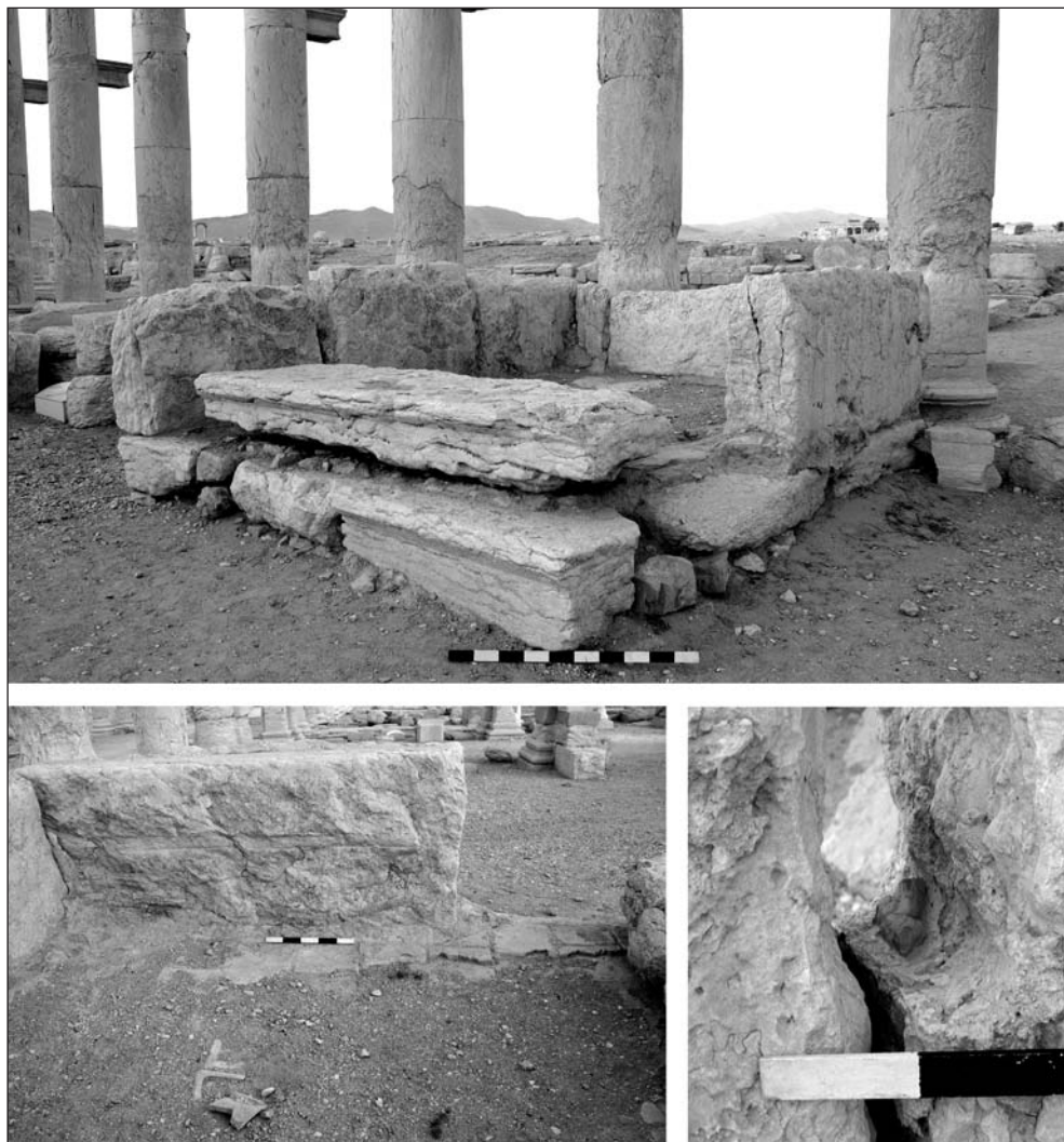
Fig. 6. Water tank near the Theatre, probable sabil : top, view of the structure from the southeast; bottom left, remains of the floor inside the tank against the east wall; right, clay pipe running through the west wall (seen from outside), probably part of a tap
