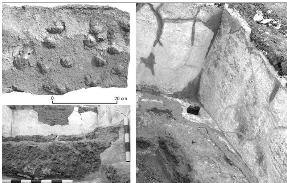
Fig. 5. Gypsum plastered steps in the ayvān (bottom left), and the wall plastering in the ayvān during conservation (right); back of a fragment of gypsum plaster showing the pock-marking of the bricks (top left)
