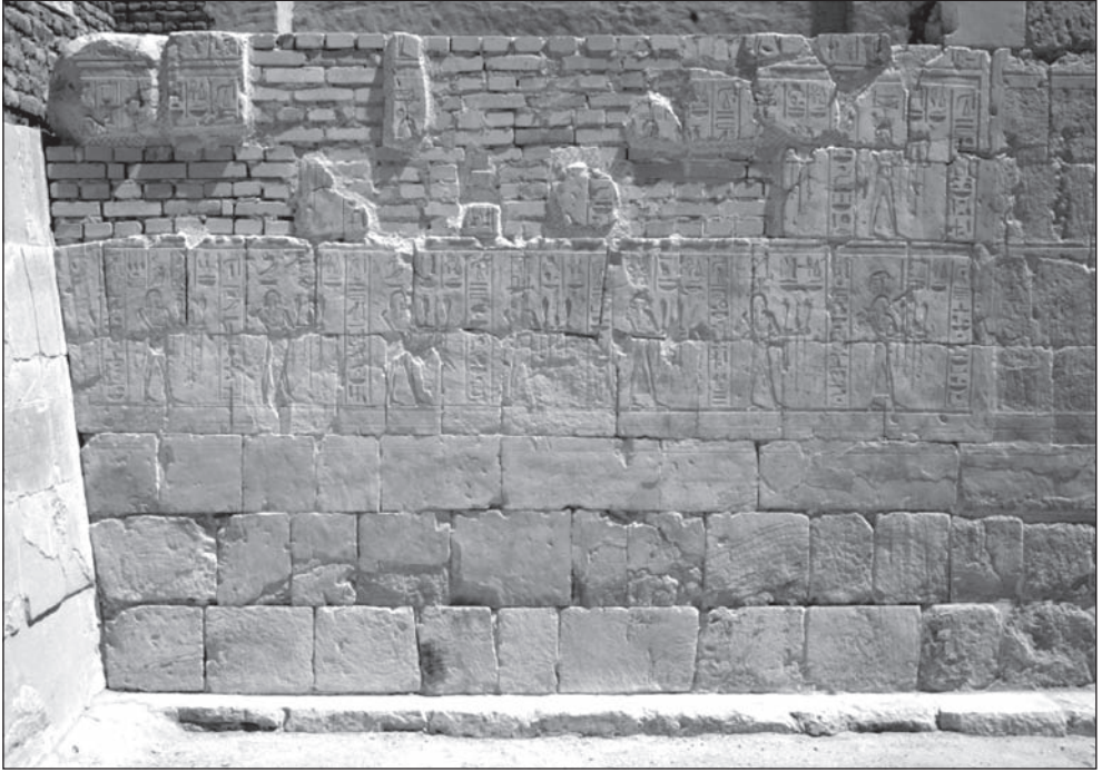
Fig. 2A. East wall of the courtyard of the Royal Mortuary Cult Complex: rearranged restoration of blocks in the wall (Photo W. Wojciechowski)
