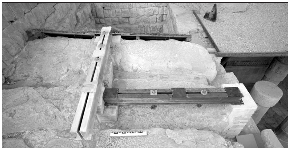
Fig. 8. Roof of the Hathor Shrine vestibule reinforced with a steel construction (Photo W. Wojciechowski)
