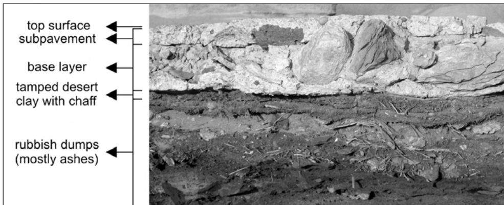
Fig. 3. Cross-section through the pavement in unit B.22 (Photo S. Maślak)
