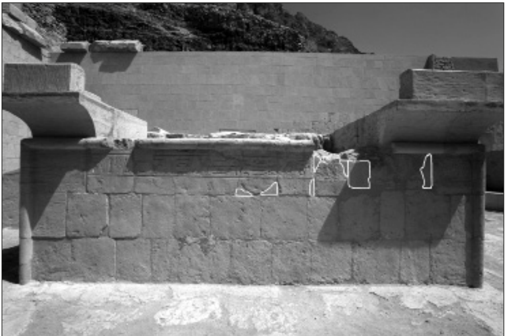
Fig. 2. South face of the Sun Altar, restoration with new limestone (outlined in white) (Photo M. Jawornicki)
