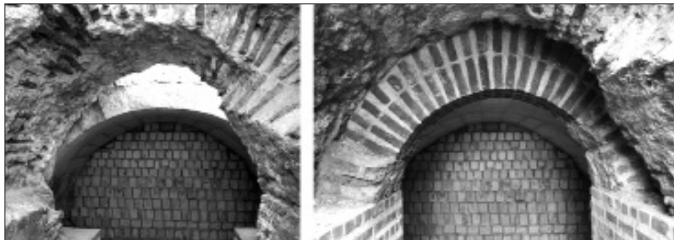
Fig. 13. One of the restored vaults giving access to the furnaces in the baths, before (left) and after restoration (Photo A. Pisarzewski)
