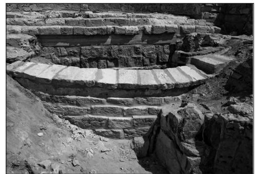
*Fig. 3. Outer wall of the kiln, inboard face (left) with new mud-brick infill and brick and stone coping, and outboard face (right) with new retaining wall and coping (Photo Jack M. Kucy)*
