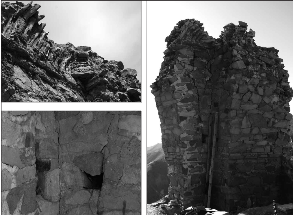
Fig. 3. Masonry in the southern corner of the chahar taq, including close up of the squinch (top left) and of the putlog holes (bottom left) (Photo B. Kaim)
