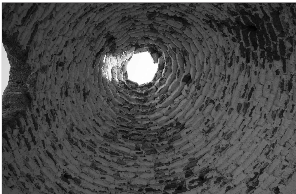
Fig. 6. Traditional qubba with cupola roof made of mud bricks and covered with plaster (top) and example of mud brick usage in cupola roof construction, both from Qaramel village (Photos R.F. Mazurowski)
