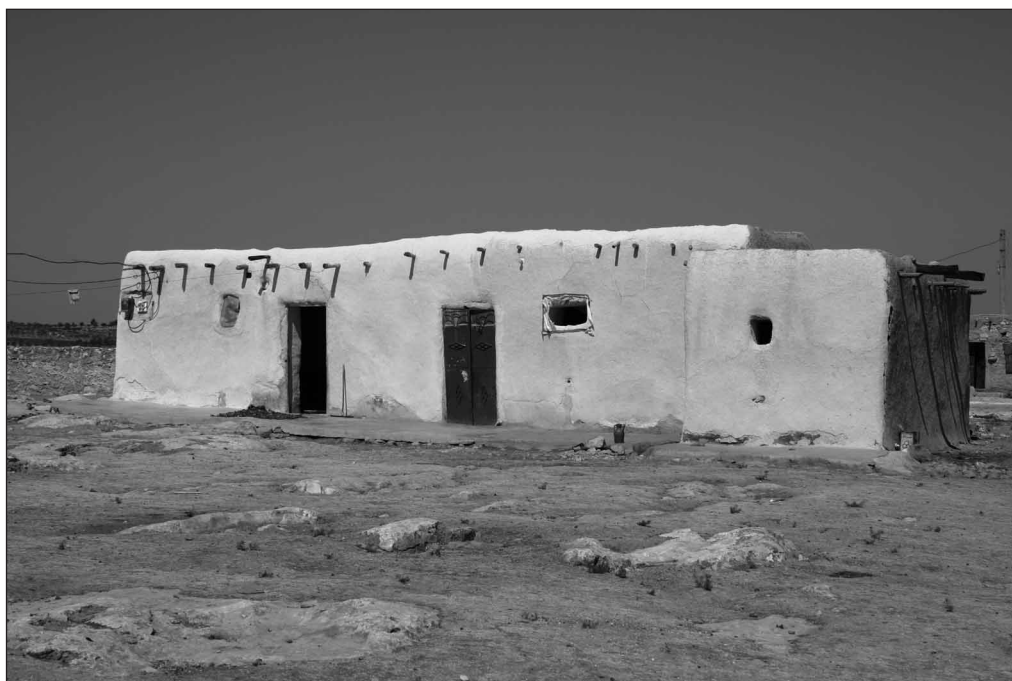
Fig. 4. Traditional Arabic house made of pisé . Qaramel village (Photo R.F. Mazurowski)
