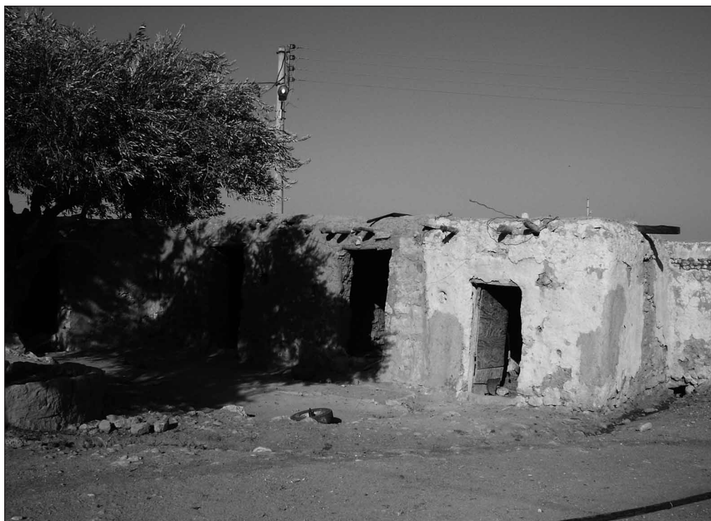
Fig. 3. Storage buidings made of pisé. Qaramel village (Photo M. Białowarczuk)
