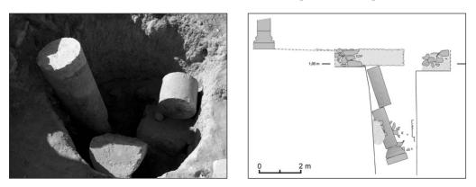
Fig. 2. The cistern in the northwestern corner with the collapsed column and other architectural elements in it (Photo M. Gawlikowski; drawing M. Wagner)
