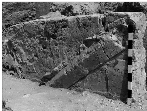
Fig. 8. Springing of stone vault under staircase in House FB, view from the south (Photo G. Majcherek)
