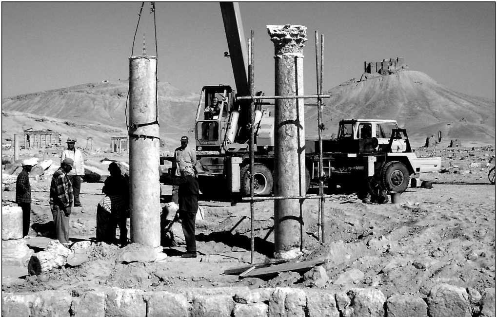
Fig. 5. Raising of the columns in the atrium of Basilica III (Photo M. Gawlikowski)
