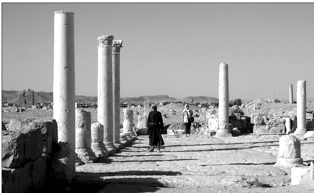
Fig. 7. The restored atrium of Basilica III, seen from Church Street (Photo M. Gawlikowski)
