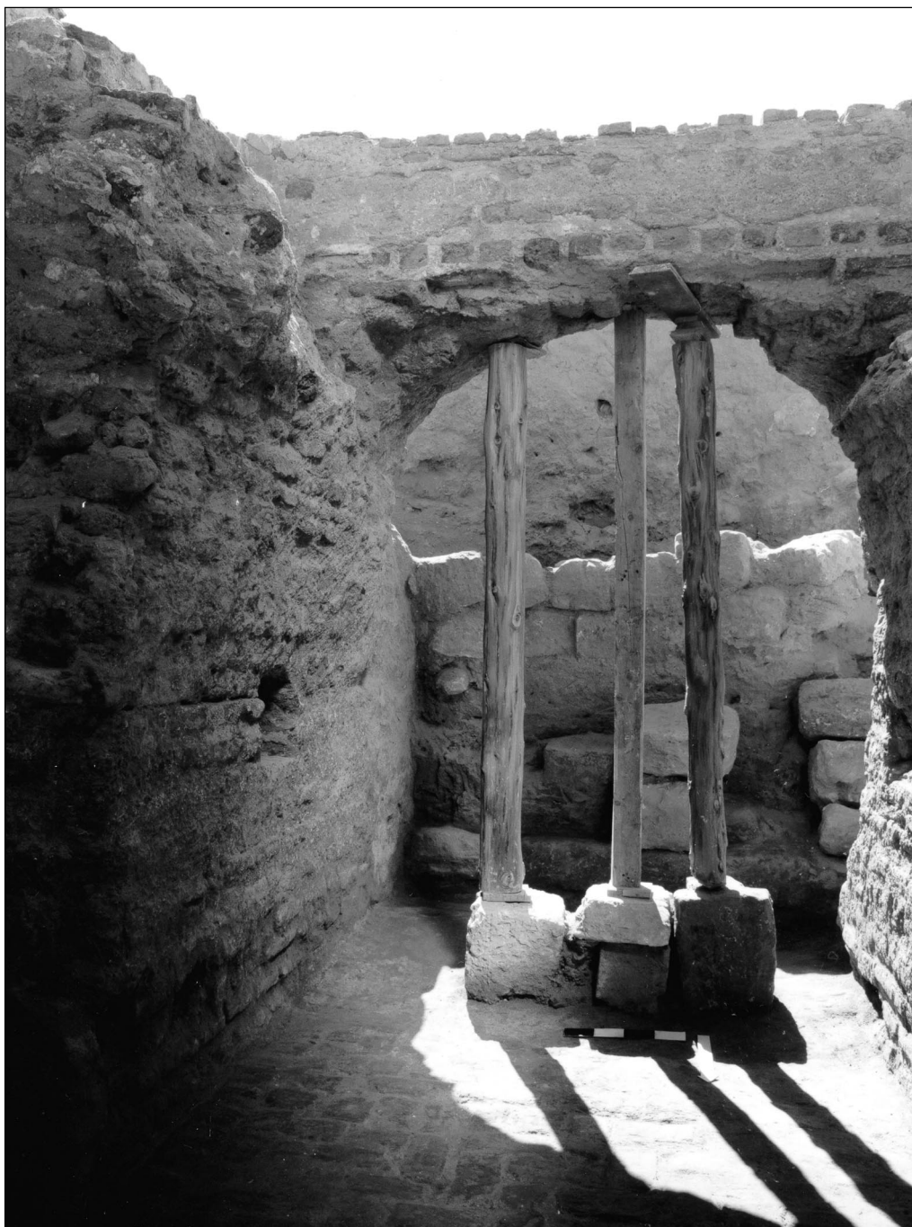
Fig. 13. Wooden support under vault of the entrance into the space under chamber A2, view from the north (Photo T. Kalarus)
