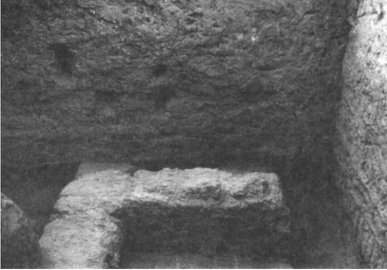
Fig. 4. House A.106. South wall founded on earlier structures (House A.111). Photo W. Godlewski.
